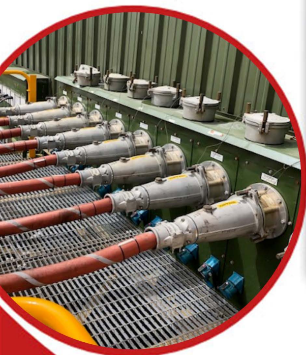
15kV, 800A Shielded Couplers in service in Latin American gold mine
