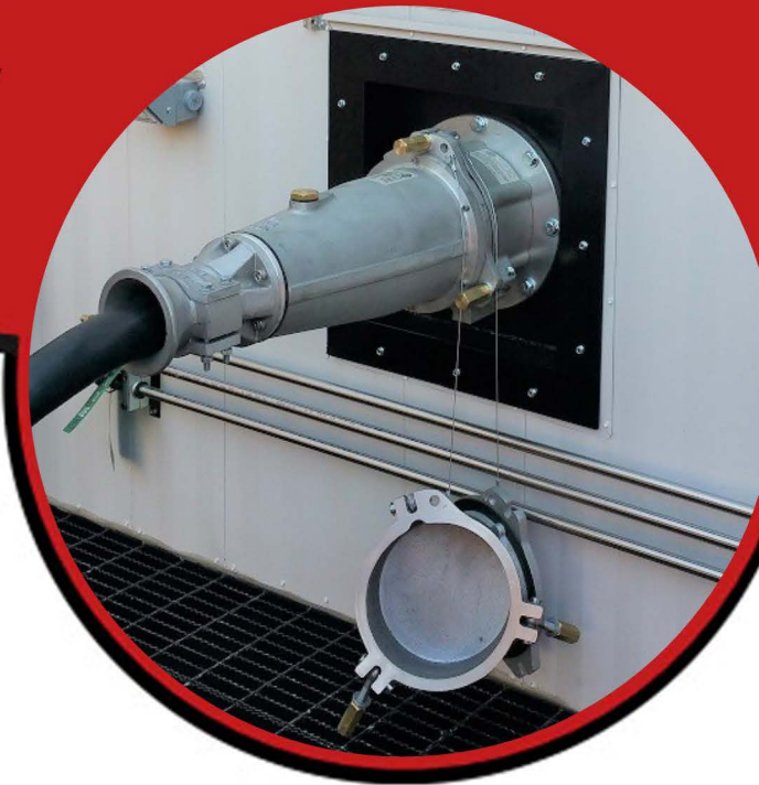
15kV, 600A Male Shielded Couplers in service on MCS manufactured Cable Repair Facility
